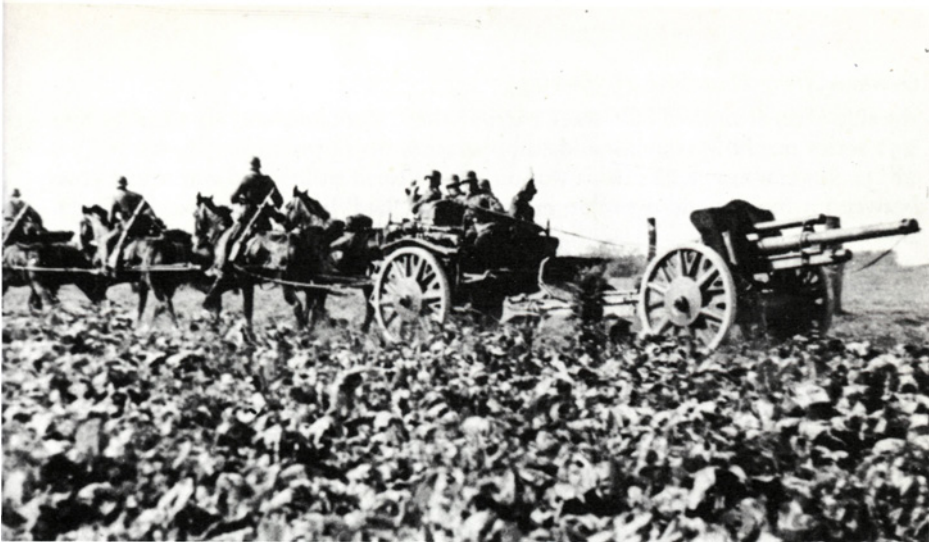
48. An old-pattern leFH18 in 'horse-drawn' guise. Note the box trail, the crew-carrying limber and the invariable rider on each offside horse. (HU 3894)
